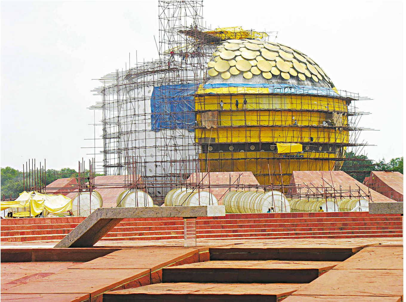
Replacing the discs in 2005, after renewing the waterproofing
