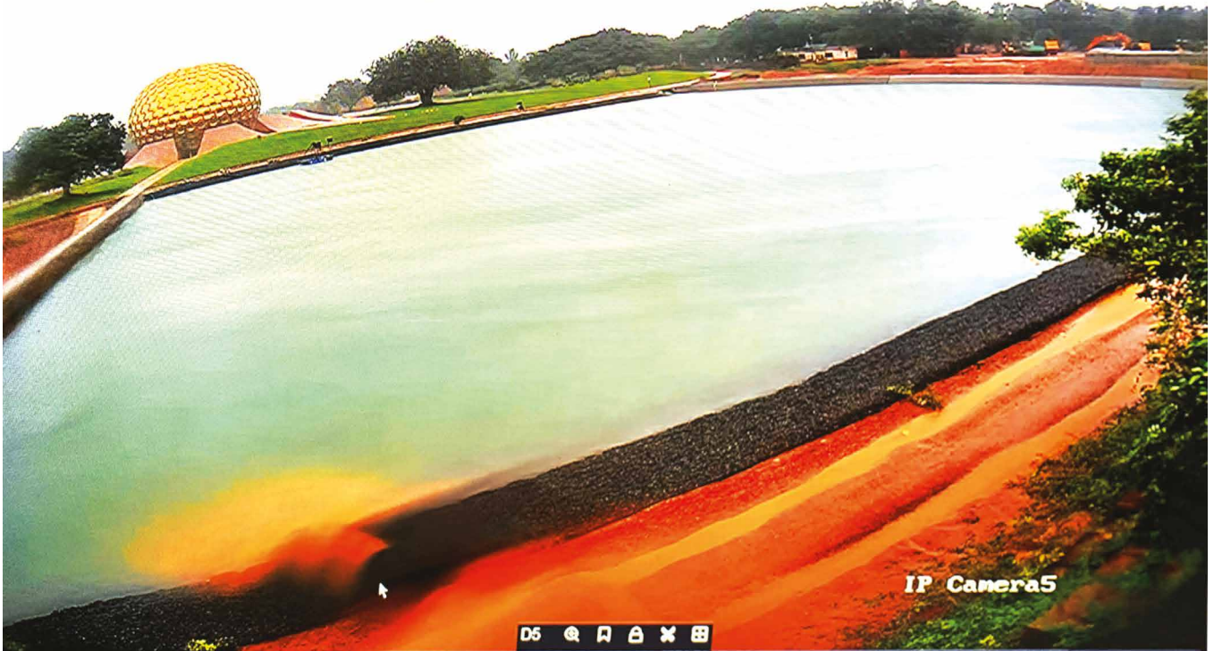
The Matrimandir lake, section 1, completely filled by the rains of cyclone Fengal on 30 November 2024, just before the left end wall slid open.
